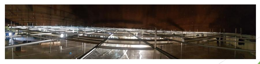
Installation of Aluminium internal floating roofs 6pcs - diameter 36m
