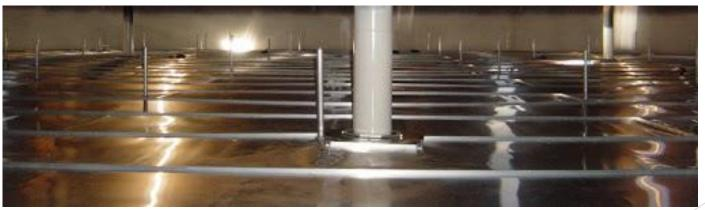
Installation of heating coils in a tank - volume 25.000m3
